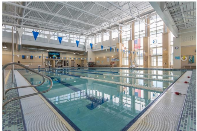
FIGURE 17 GARRETT COLLEGE AQUATIC & RECREATION CENTER POOL
