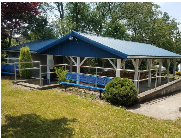
FIGURE 13 PAVILION AT DEER PARK
