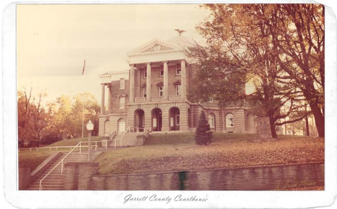
GARRETT COUNTY COURTHOUSE COMMISSION - 1907
