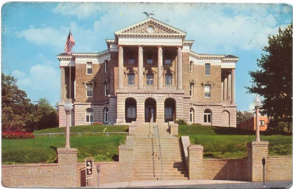
GARRETT COUNTY COURTHOUSE VIEW FROM THIRD STREET PRIOR TO SHERIFF'S DEPARTMENT AND JAIL ADDITION
