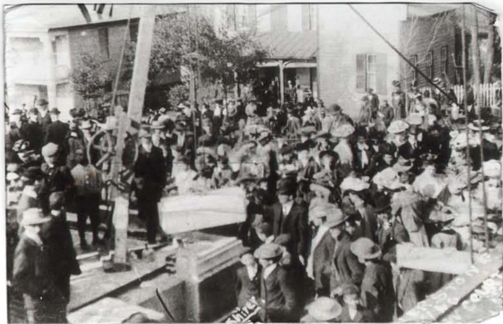
LAYING THE CORNERSTONE FOR THE GARRETT COUNTY COURTHOUSE.
