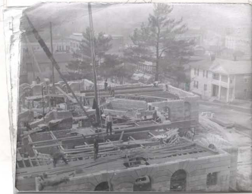
CONSTRUCTION OF THE FIRST FLOOR OF THE COURTHOUSE.
